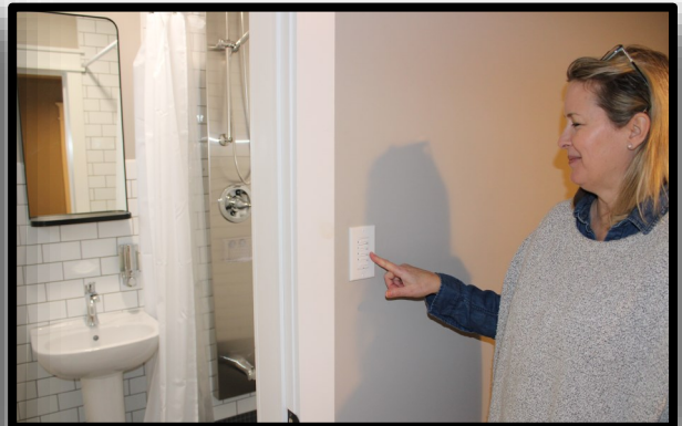
Above: Marinka Molson demonstrates the switch panel that operates the heated bathroom floor.
