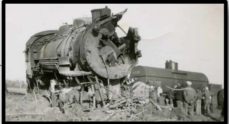
Above: In this photo from the Sarnia Observer, a front view of north-bound Engine No. 751 shows the massive breach that was created during its collision with the tank cars of the second train. Workmen are seen beginning the task of untangling the wrecks so rail service can resume.
