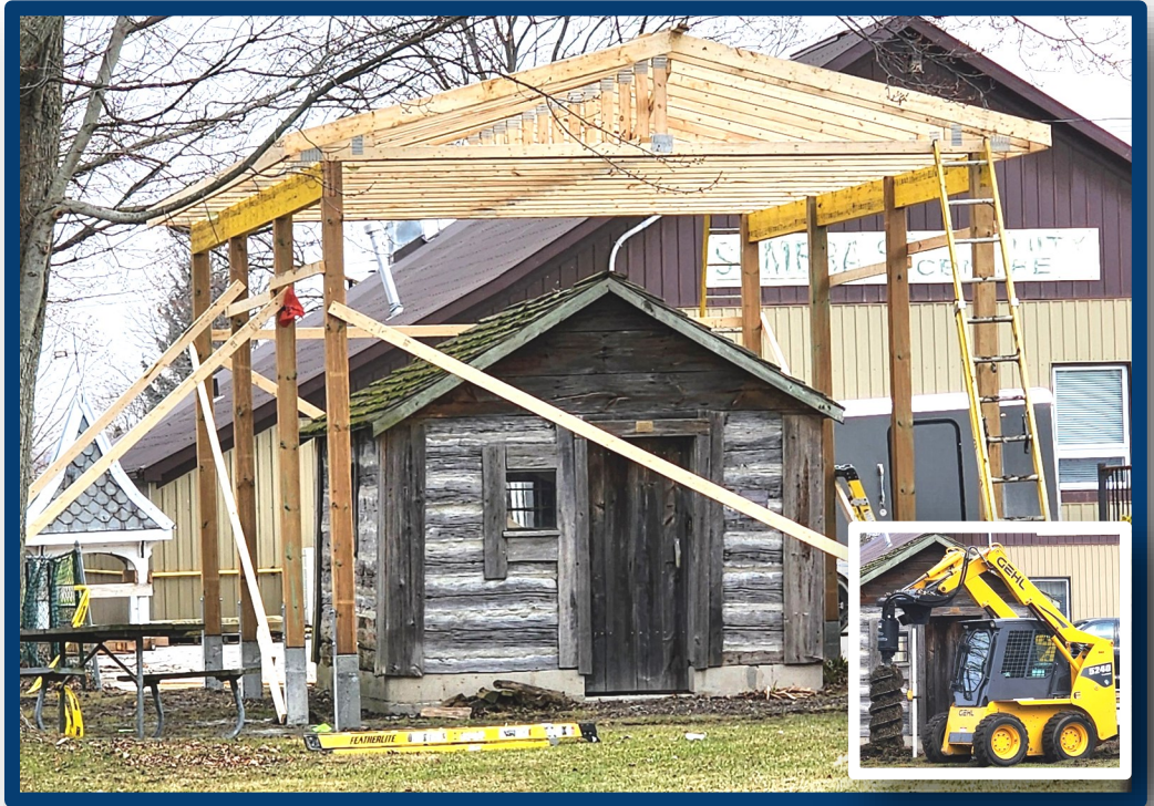
Above: The new pavilion under construction.
